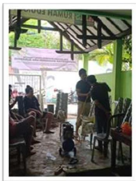
Gambar 4. Proses Pengecatan Pipa Paralon
