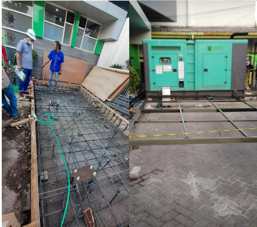
Gambar 5. Proses Pengerjaan Pondasi Genset RSI Ahmad Yani
